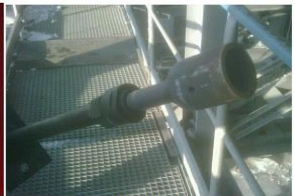
Ceramic pilot after two years in operation
