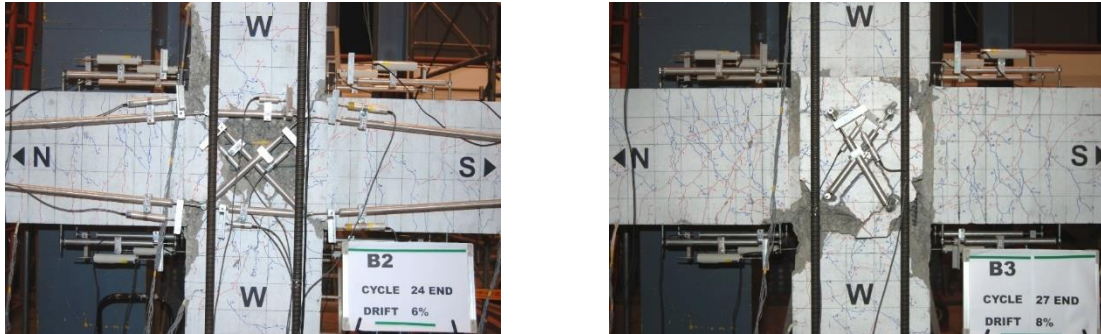
Figure 6. Final damage patterns of Specimen B2 and B3.
