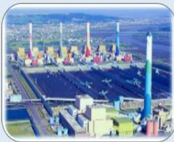
Coal-Fired Power Plant
