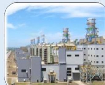
Combined-Cycle Power Plant
