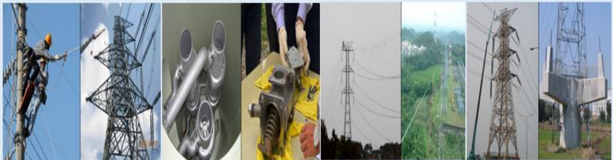
Replacement of Insulators and Towers
