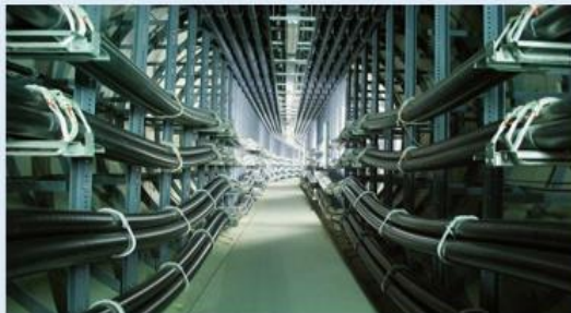
345kV Underground Cables
