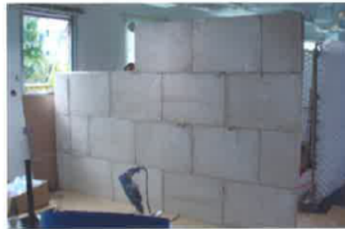
圖4 石膏牆 (資料來源：香港綠色建築協會) Figure 4 Gypsum block wall (Source: Hong Kong Green Building Council)
