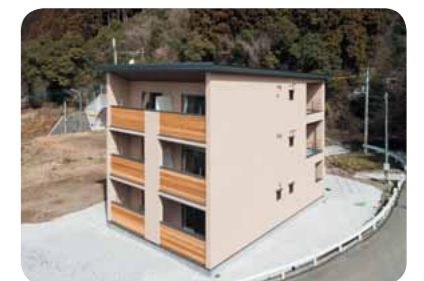
A three-story company dormitory using CLT (Otoyo Town, Kochi Prefecture)
