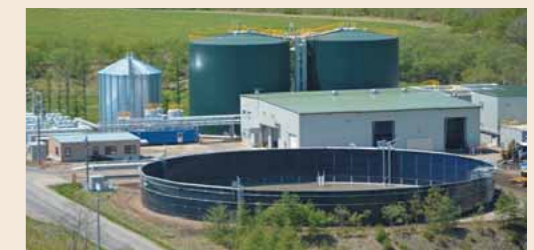
Biogas power generation facility
