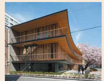
Osaka Mokuzai Nakagai Kaikan (Osaka City, Osaka Prefecture): Fire-resistant structure Photo: T. HAHAKURA
