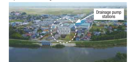
Implement water drainage measures
