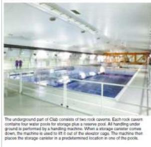
The underground part of Clab consists of two rock caverns. Each rock cavern contains four water pools for storage plus a reserve pool. All handling underground is performed by a handling machine. When a storage canister comes down, the machine is used to fit it out of the elevator cage. The machine then places the storage canister in a predetermined location in one of the pools.
