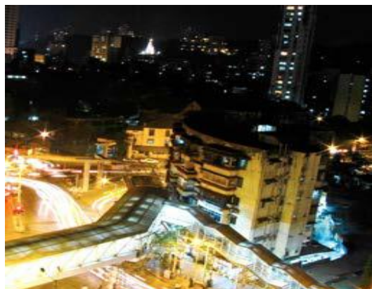
Power grid expansion, Maharashtra
