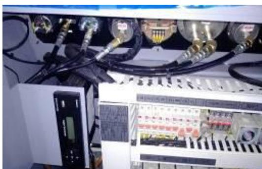
A photograph of the same terminal block after improvement. The wires are now organized into neat bundles, secured with black zip ties. The bundles are clearly labeled with white tape, and the overall wiring is much more orderly and secure.                         |
