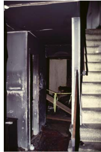
First Floor Hallway
