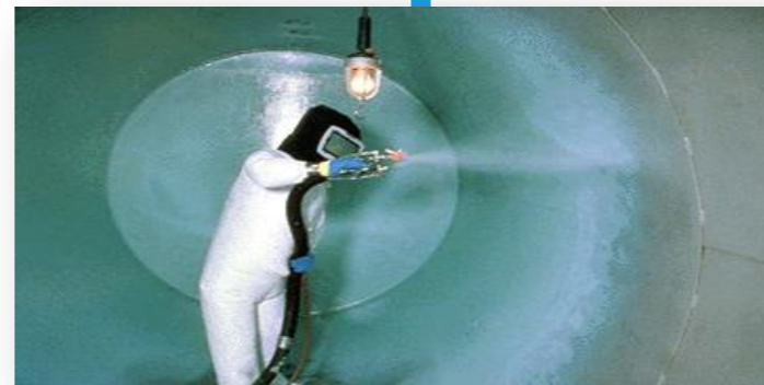
2. Execution of the first metal coating
