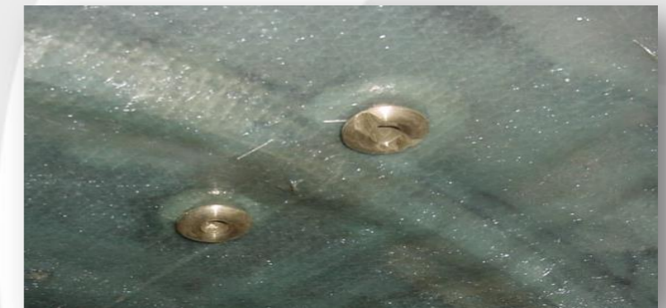
3. Install the fittings for monitoring device of the interspaces
