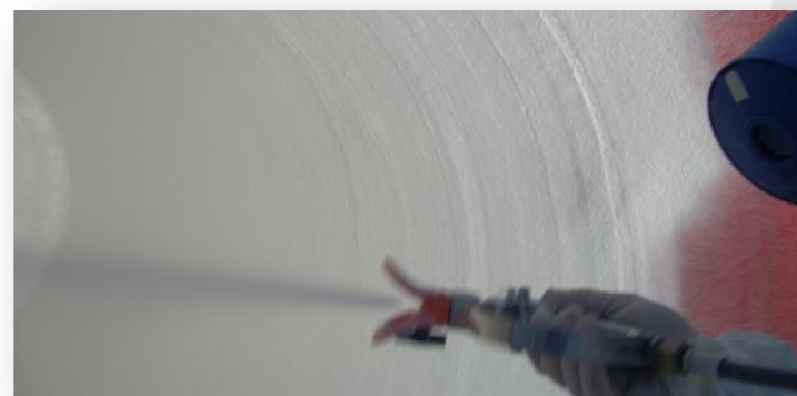
5. Realization of the 2° coating of the double wall
