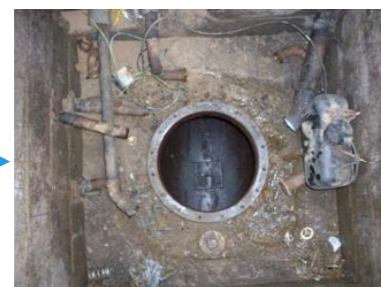
Tank cleaned and in Gas-Free
