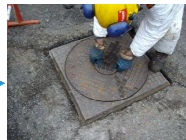
Re-install the tank LID and close the pit
