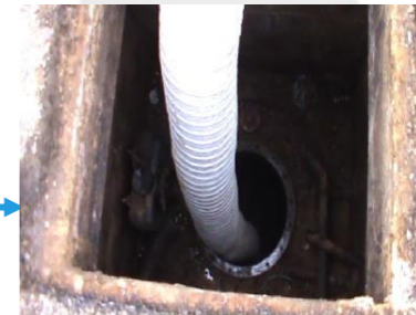
Venting the tank
