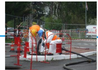
Cleaning and Gas-free the pit
