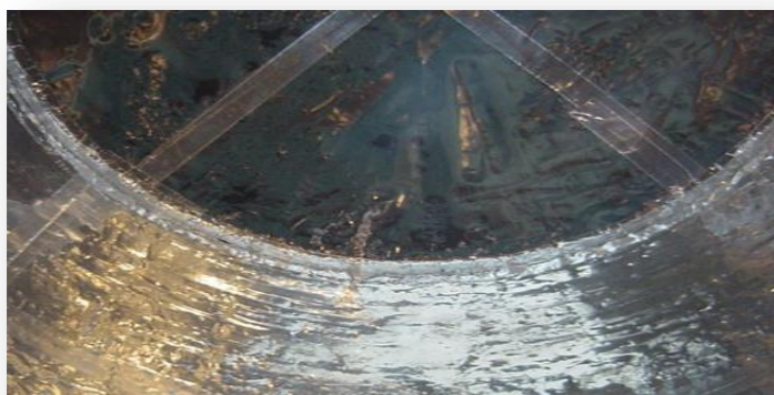
4. Realization of the 1° coating of the double wall
