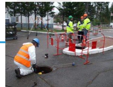
Disconnecting piping and opening the LID
