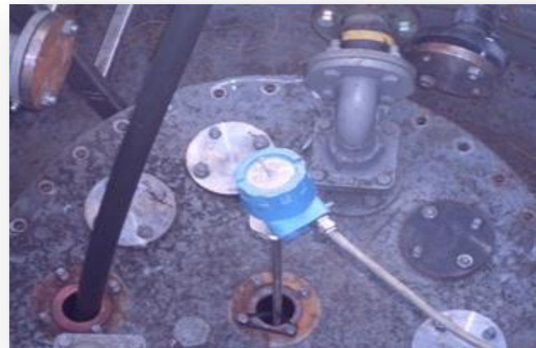
Magnetostrictive level probe
