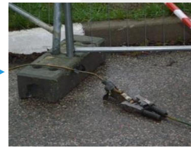
Connect all system to ground cable
