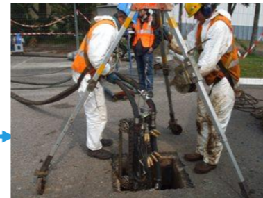
Removing BRUCO System
