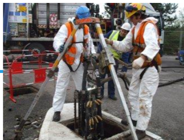
Place the BRUCO System inside the pit
