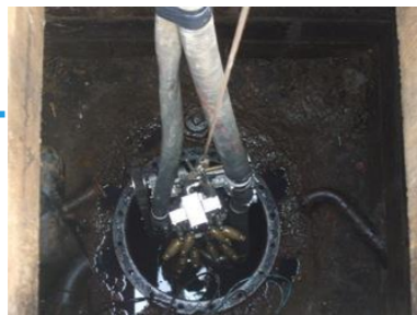
Place the BRUCO System inside the tank
