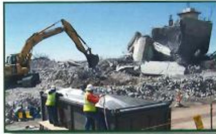
Building demolition at the Engine Maintenance, Assembly and Disassembly Facility.
