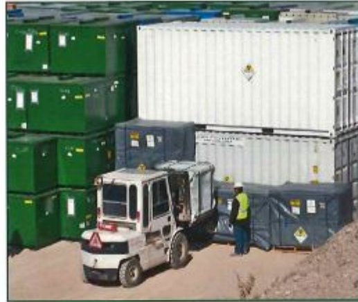
Waste packages are positioned in a disposal cell at the NNSA Area 5 Radioactive Waste Management Site
