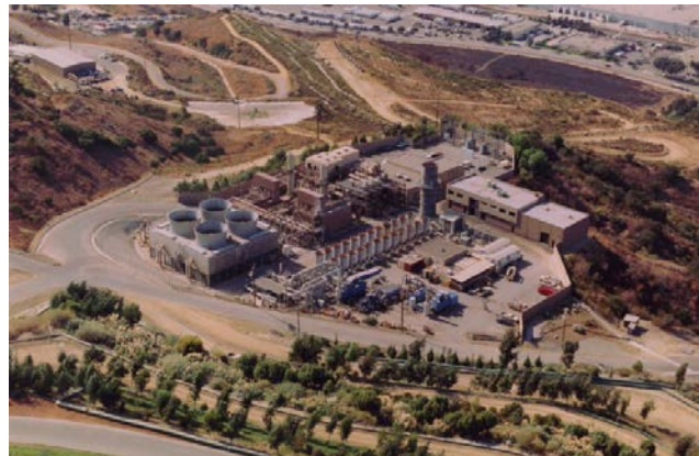
Figure 3 - The Los Angeles County Sanitation District (LACSD) in California has operated a 50 megawatt (MW) landfill gas energy project at its Puente Hills Landfill since 1985, producing electricity for customers throughout Los Angeles.
