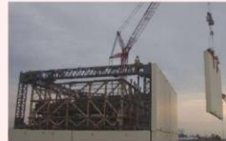
<Dismantling of wall panels>
