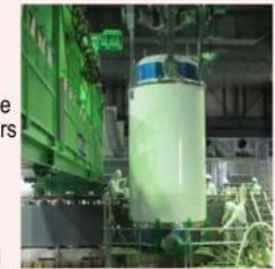
Fuel removal status
