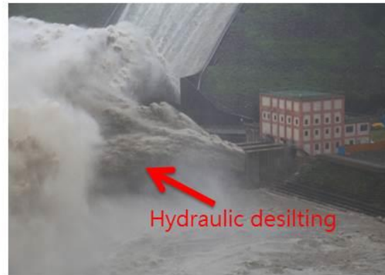
hydraulic desilting in Typhoon Soudelor
