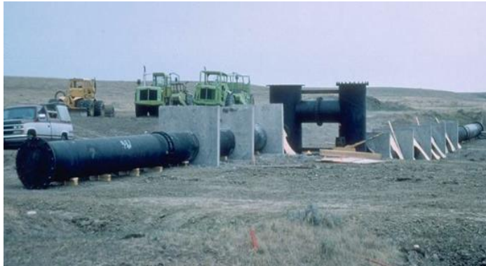
Anita Dam 渠道施工
