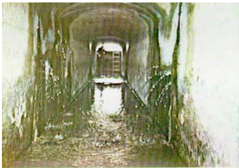
Photo 19. Deer Flat Dams - Deer Flat Caldwell Canal outlet-works conduit, looking toward the downstream end. Note the seepage at the sides of the conduit. 3-18-86
