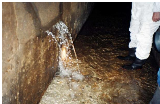
Photo 19. Deer Flat Dams - Deer Flat Caldwell Canal outlet-works conduit, looking toward the downstream end. Note the seepage at the sides of the conduit. 3-18-86
