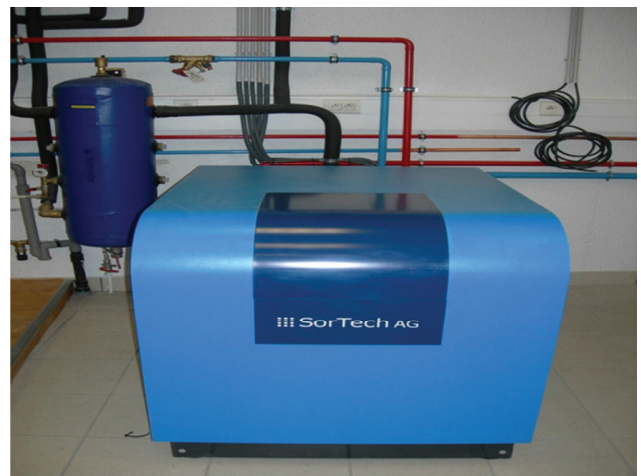
Fig. 5: adsorption refrigeration machine
