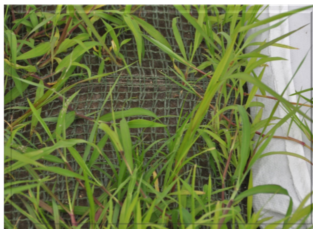
Figure 4. Erosion control mats in the Kamisaigo River.
