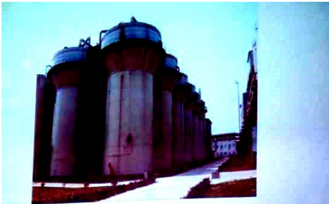
Commercial ethanol production by the flocculating yeast (200, 000 t/y).
