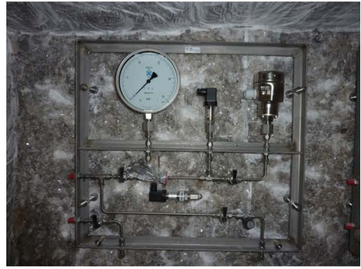
Pressure gauge + separator
