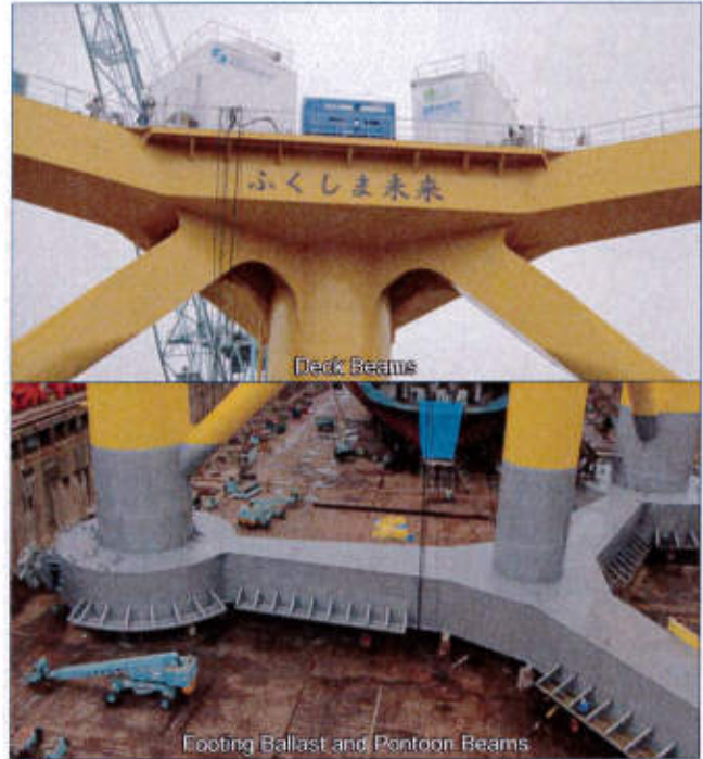
Footing Ballast and Pontoon Beams
