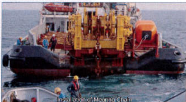
Installation of Mooring Chain
