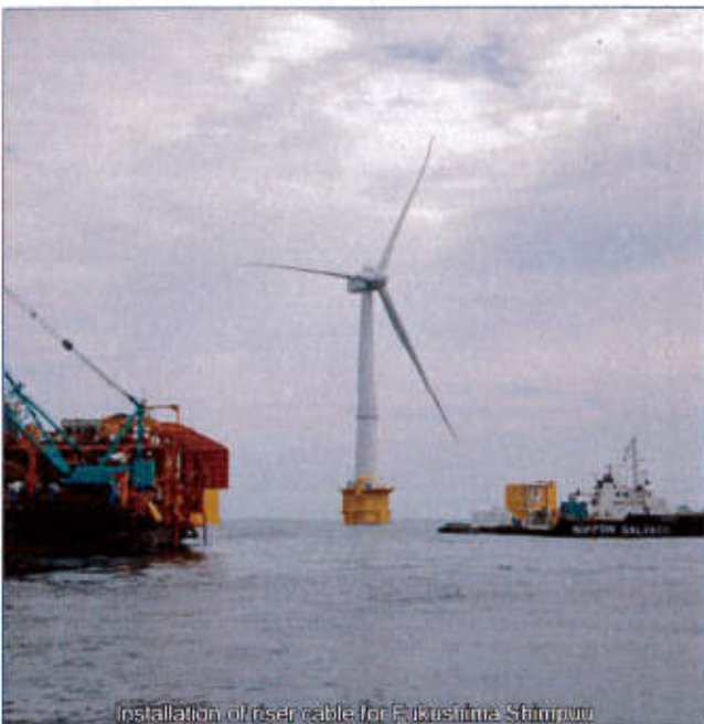
Installation of riser cable for Fukushima Shimpuu
