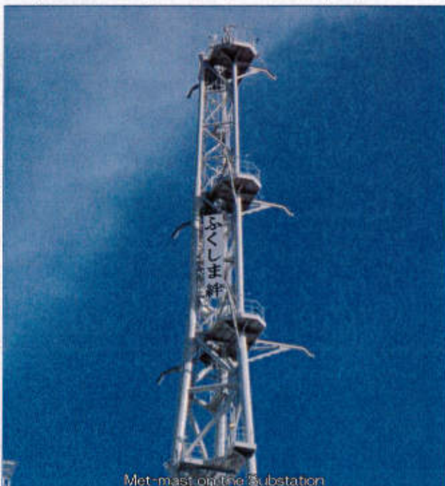
Met-mast on the Substation
