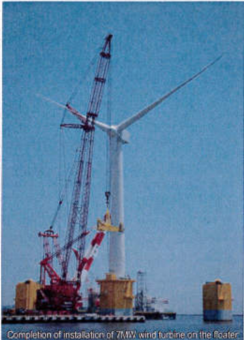
Completion of installation of 7MW wind turbine on the floater
