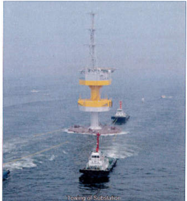
Towing of Substation
