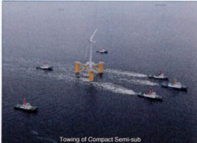
Towing of Compact Semi-sub
