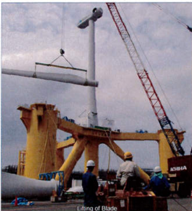
Lifting of Blade
