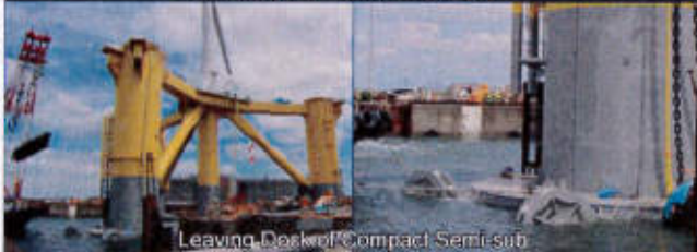
Leaving Dock of Compact Semi-sub
