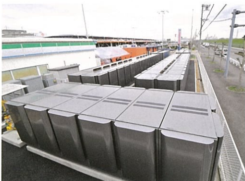
Fuel cell system of 1.2 megawatt solid oxide fuel cell(or SOFC) The service started in March 2015
