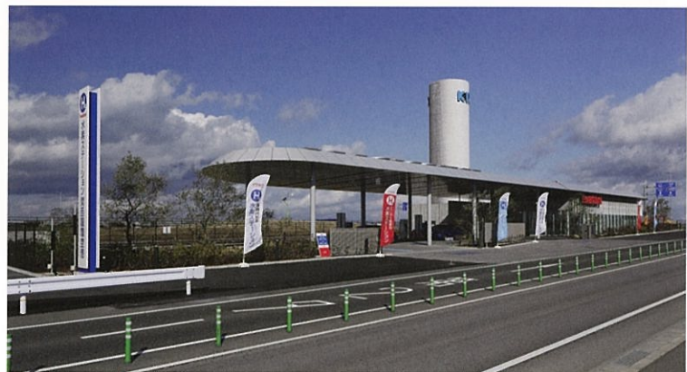
Iwatani Hydrogen Station in Kansai International Airport (Open in January 2016)
