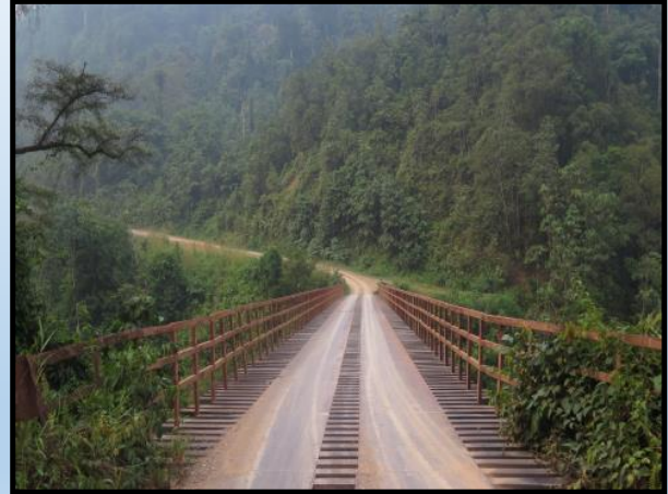
Steel bridge leading to Long Napir
