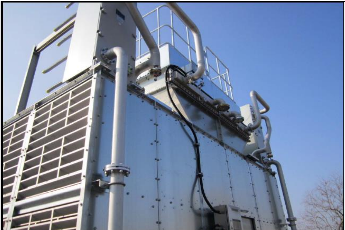
三宮變電所用密閉型冷卻水塔(TOWEREX TYPE)
