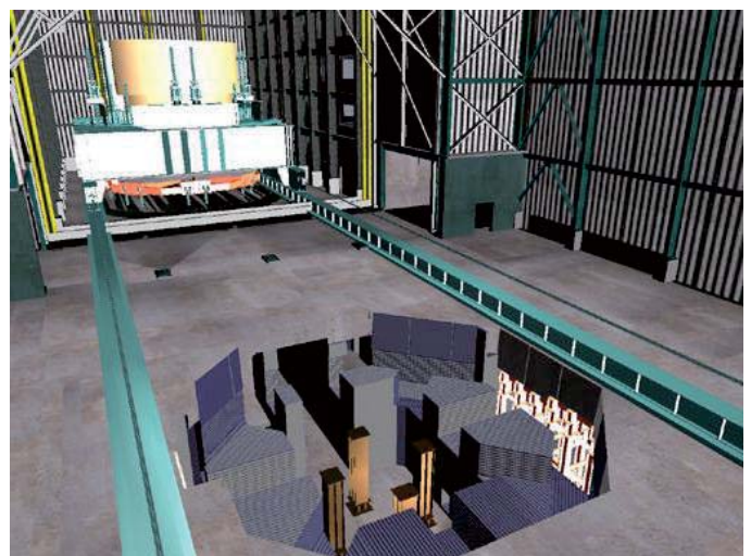
TRR was stopped running and executed one piece removal operation
