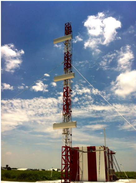
The new installed ILS/DME for Runway 20 in Magong Airport
