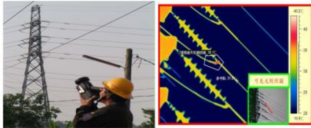
Infrared ray thermal measurement
