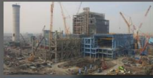
Talin Coal-Fired Power Project (1,200 MW)
