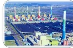
Coal-Fired Power Plant
