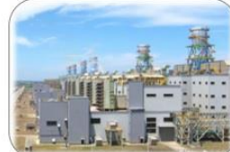
Combined-Cycle Power Plant
