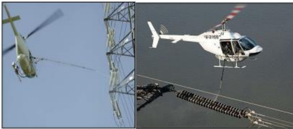
Using helicopter for insulator washing
