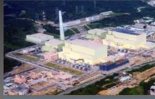
Lungmen Nuclear Power Project (2,700MW)
