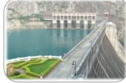
Hydro Power Plant
