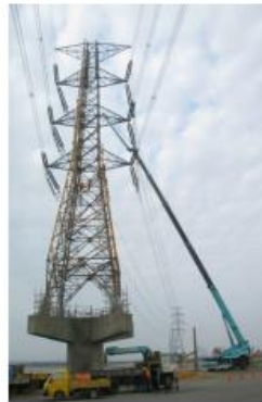
Outer steel construction replacing tower
