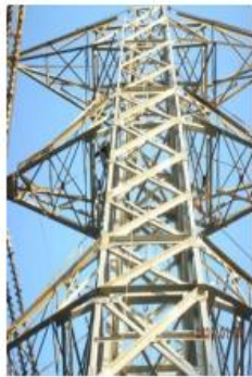
Inner Steel construction Replacing tower
