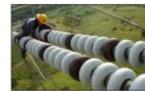
Application of Silicone Grease Coating to High Voltage Insulators)
