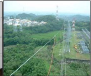
TSURIKIN method for renewing overhead transmission lines
