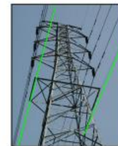
Coupling grounding wires
