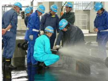
(3) Small distribution pipe leakage repair
