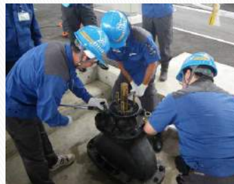
(2) Gate valve leakage repair
