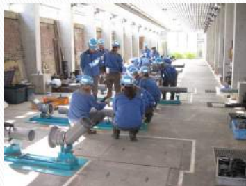
(1) Pipes connection with earthquake-resistant joints
