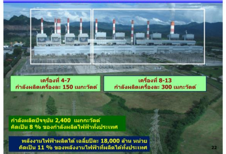
Mae Moh Power Plant Unit 4 - 13
