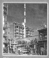
The primary purpose of this facility is to remove sulfur and metals from heavy fuel oil. Using residual oil as a feedstock, the hydrotreating process in this unit produces heavy fuel oil with even lower sulfur content, as well as middle distillates.
