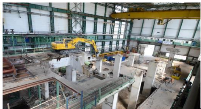
TG 22 support construction after
