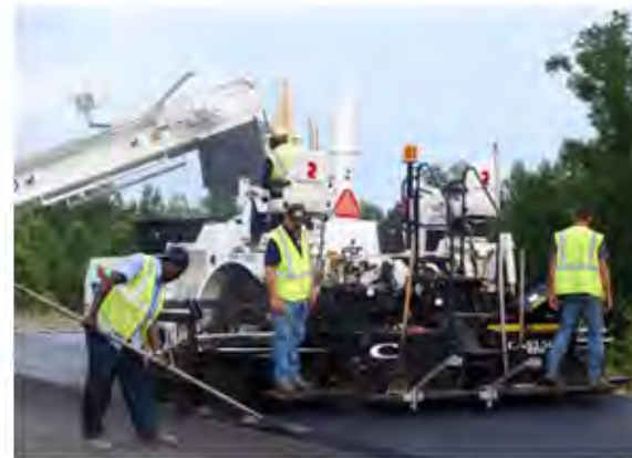
Workers lay asphalt at the NCAT track in Auburn, AL, where GTR made by Modified Asphalt Solutions is one of the top performing sections of track.
