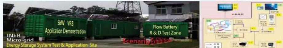
Off/On grid Integration PV~VRFB ESS with BMS/EMS
