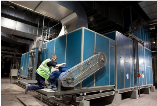
1. AHU & chiller modifications
