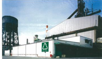
Plant equipped with facility to use plastic as blast furnace feed (Ohgishima area)
