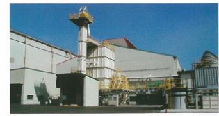
NF board manufacturing plant
