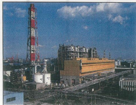
Ohgishima Thermal Power Station
