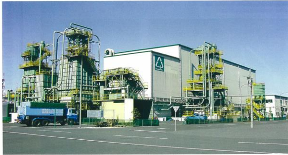
Plant equipped with facility to use plastic as blast furnace feed (Mizue area)
