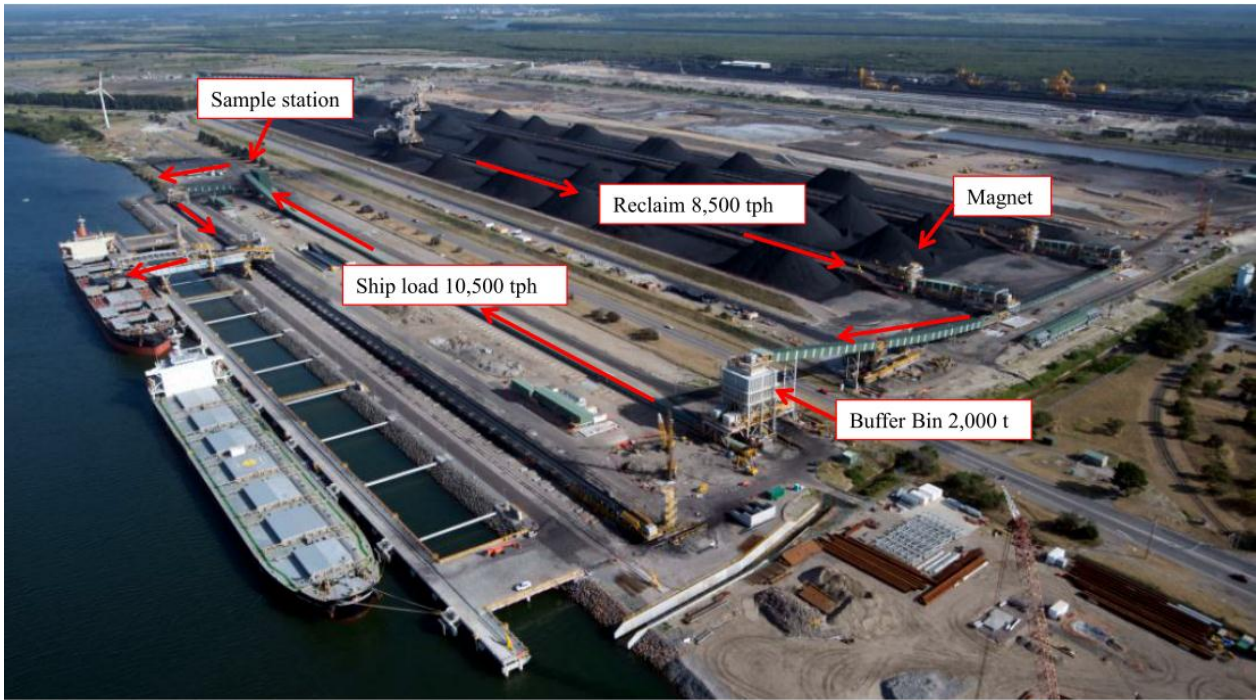
圖178 NCIG Shiploading System
