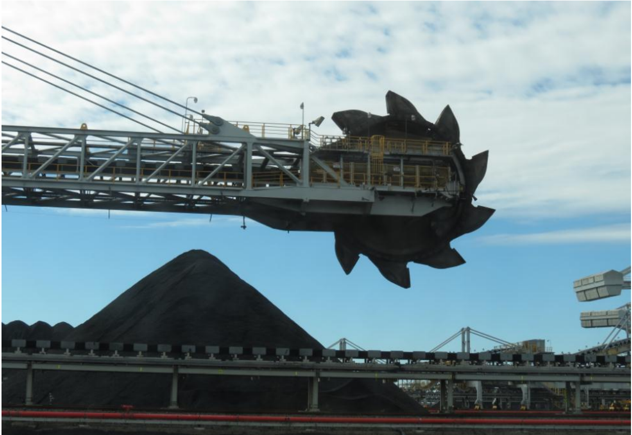
圖170 NCIG 斗輪式堆/取煤機(Bucket Wheel Stacker/Reclaimer)
