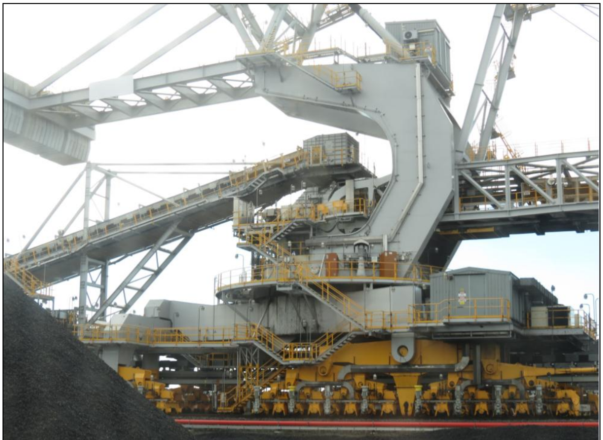
圖169 NCIG 斗輪式堆/取煤機(Bucket Wheel Stacker/Reclaimer)
