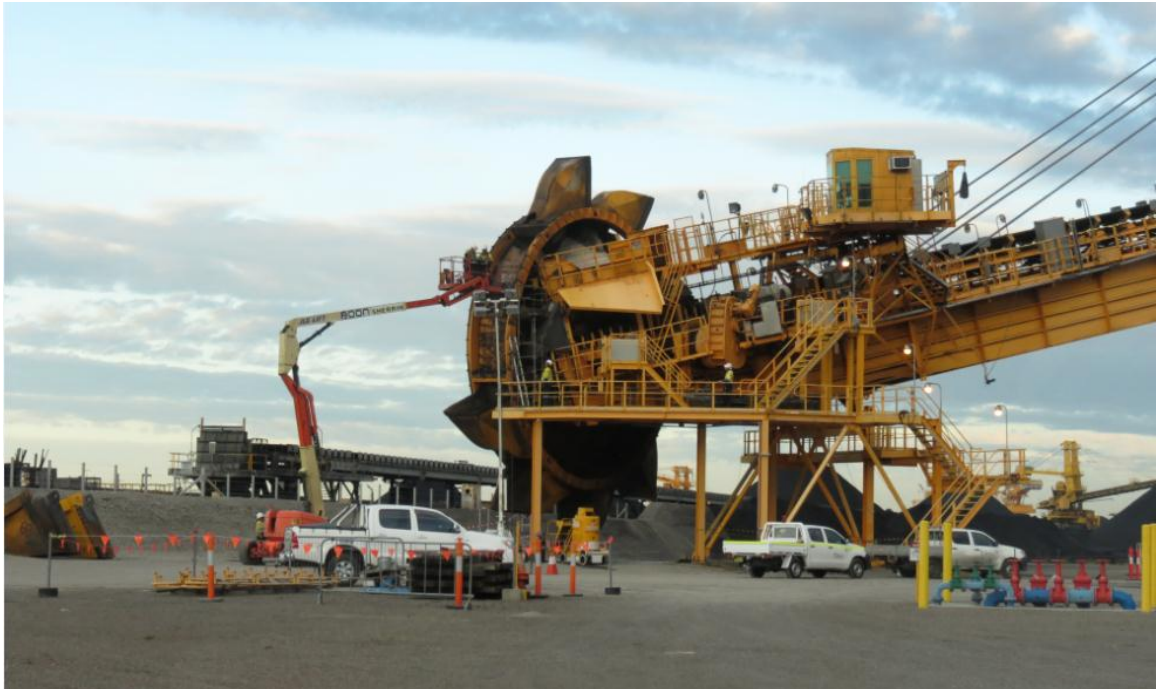
圖155 PWCS 斗輪式堆/取煤機(Bucket Wheel Stacker/Reclaimer)維修中
