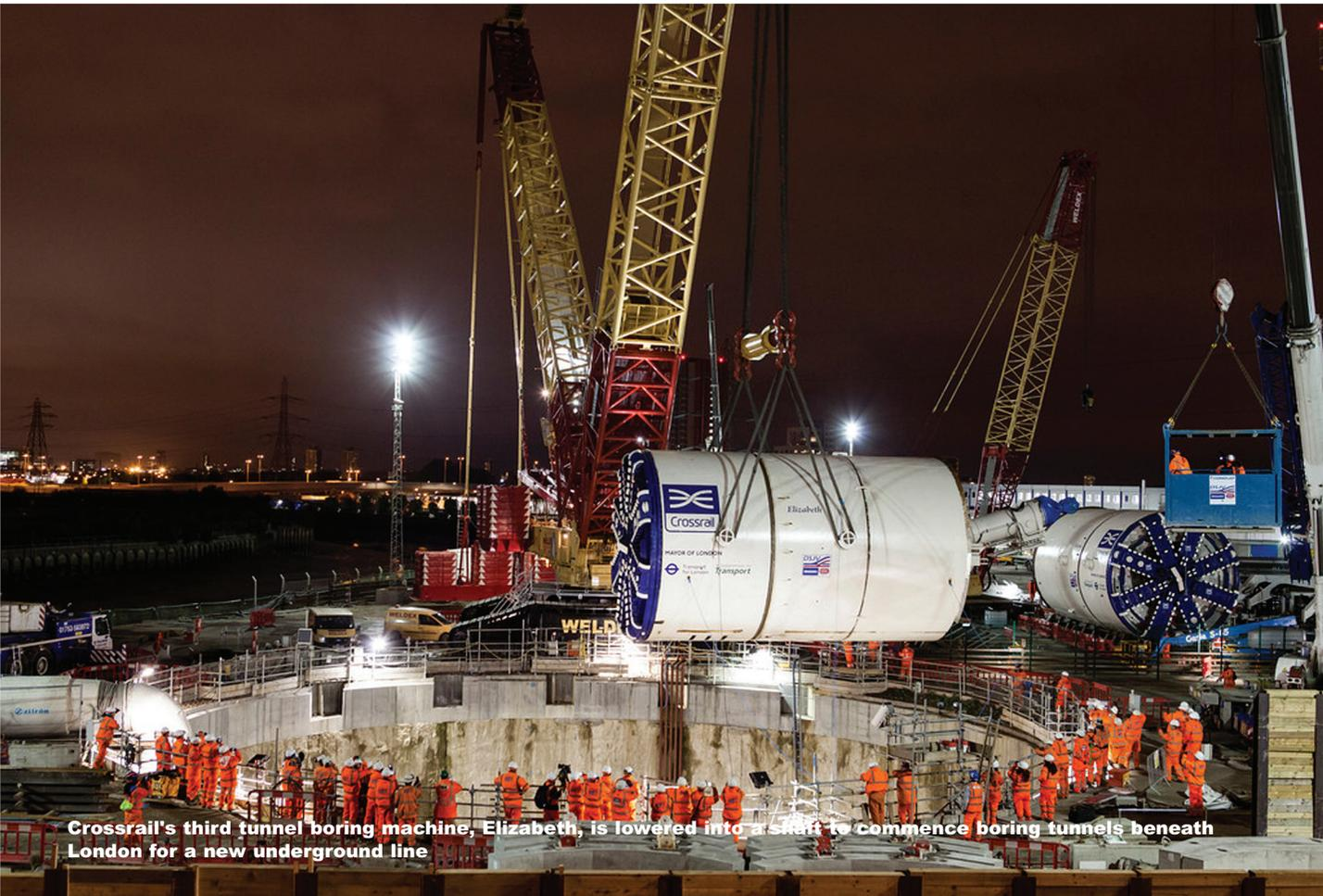
Crossrail's third tunnel boring machine, Elizabeth, is lowered into a shaft to commence boring tunnels beneath London for a new underground line
