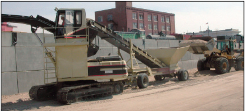
Placing backfill with a converted excavator placing conveyor
