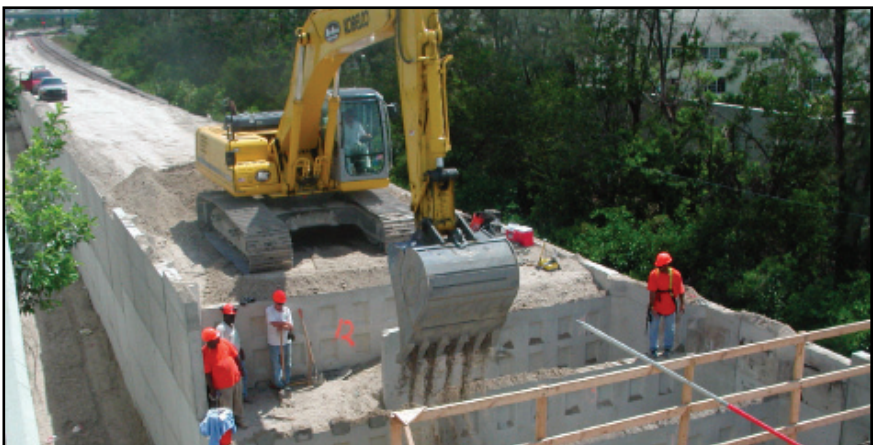
Excavator - working on top of a completed back-to-back wall
