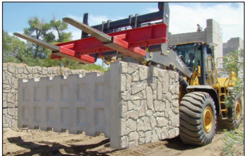
Front end loader where access is very restricted
