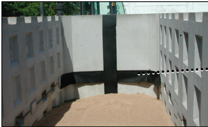
Filter fabric covering horizontal joint on the back of the face
