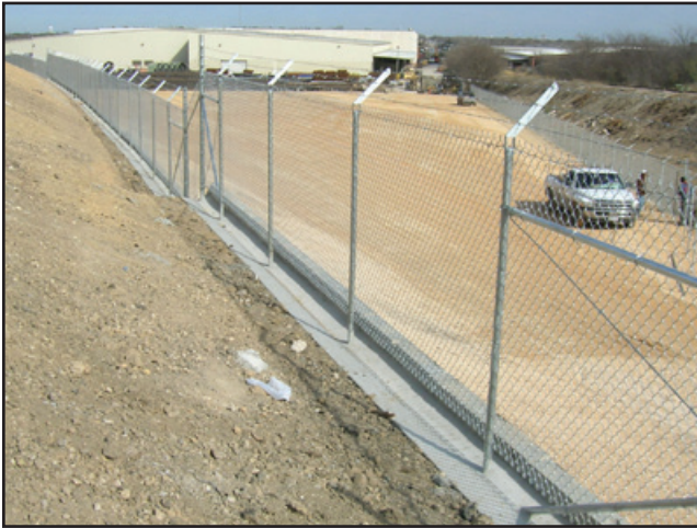
CHAIN LINK FENCE INSTALLED BEHIND THE WALL FACE:
