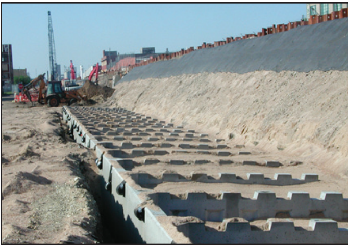
First course of units on leveling pad
