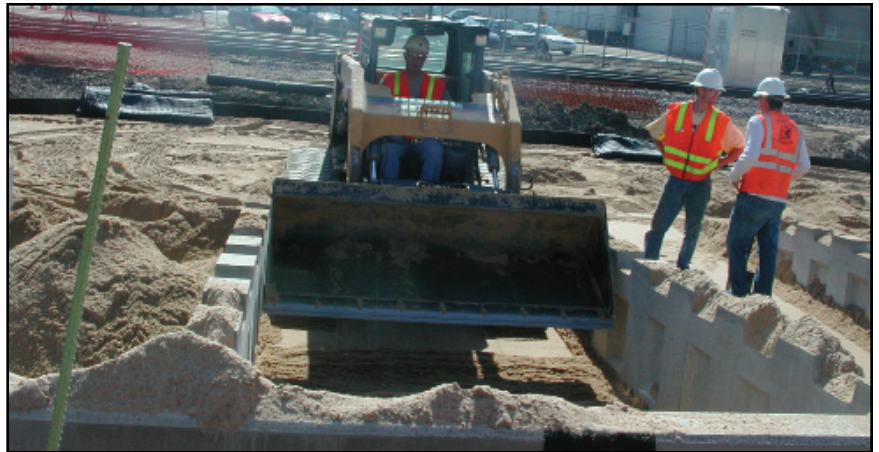
Rubber tracked skid steer loader spreading sand backfill between the stems.
