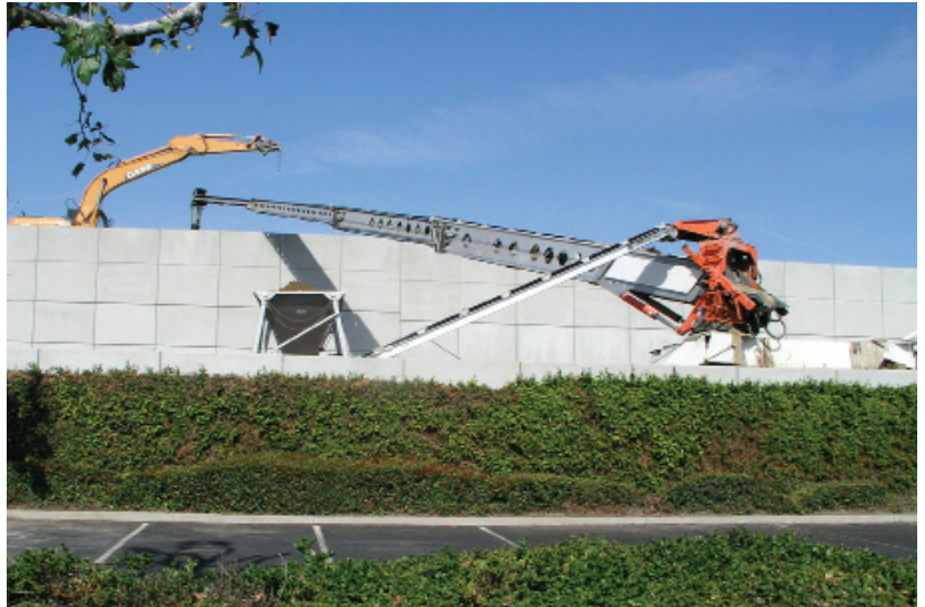
Placing backfill with a telebelt
