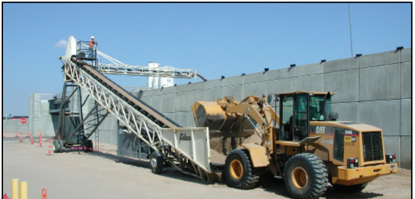
Placing backfill with a towed conveyor belt placing machine
