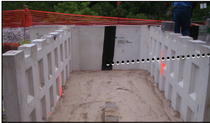
Filter fabric covering vertical joint on the back of the face
