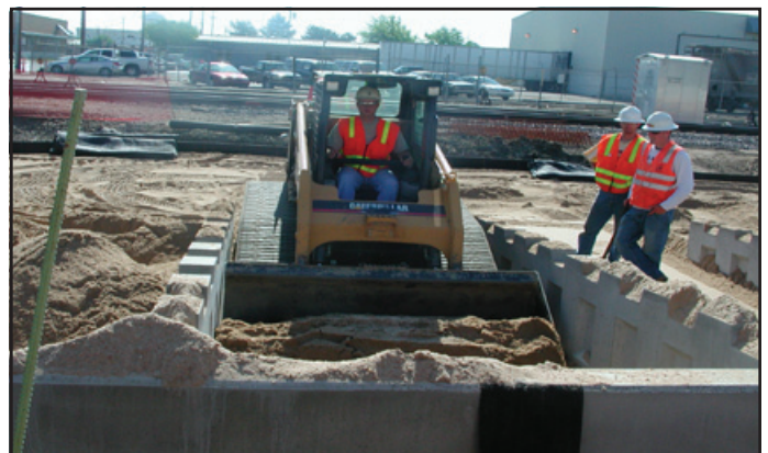
Spreading the backfill
