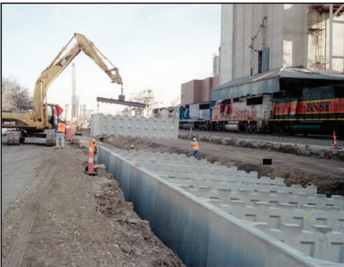
Putting units into position
