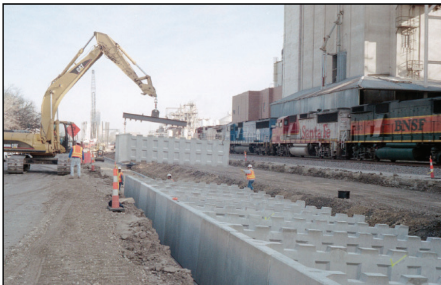
Excavator with lifting beam - working in front of the wall
