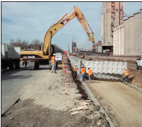
Lowering a unit into place
