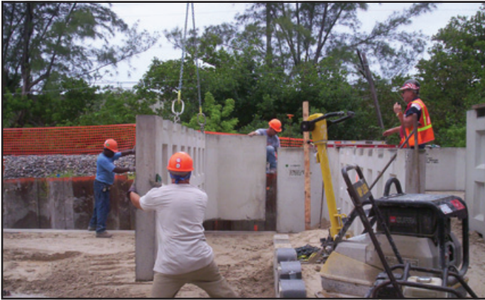
Lowering a unit into place
