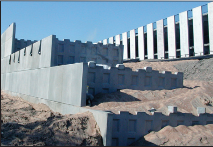
Shear keys wrapped in joint material
