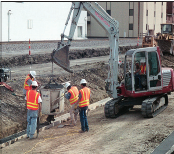
Pouring of second leveling pad
