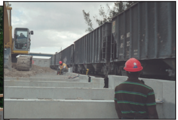
This T-WALL® bridge approach has a live train track on one side and a major highway on the other.
