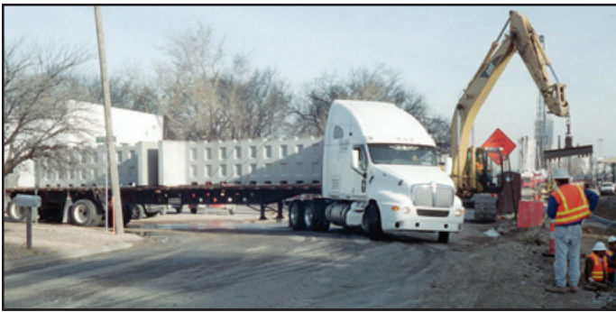
Units on truck
