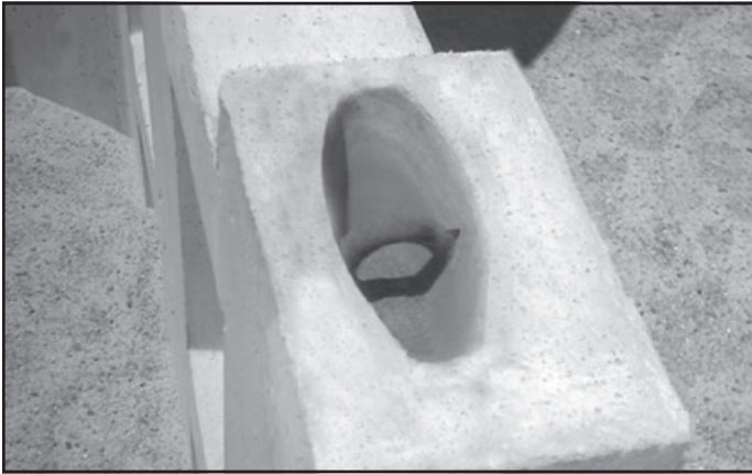
Lifting insert in stem of unit
