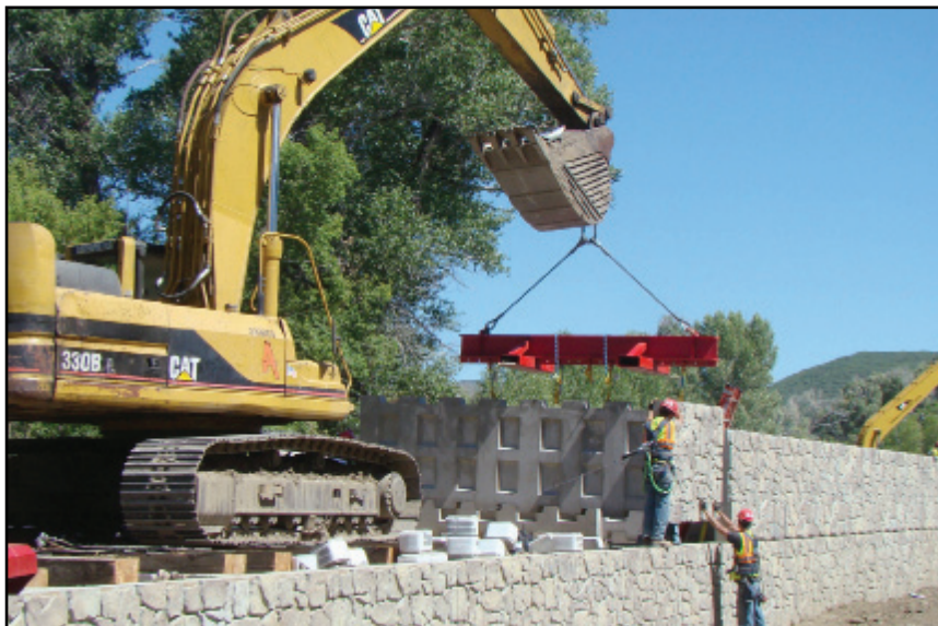
Large excavator with lifting beam - on top of back-to-back walls
