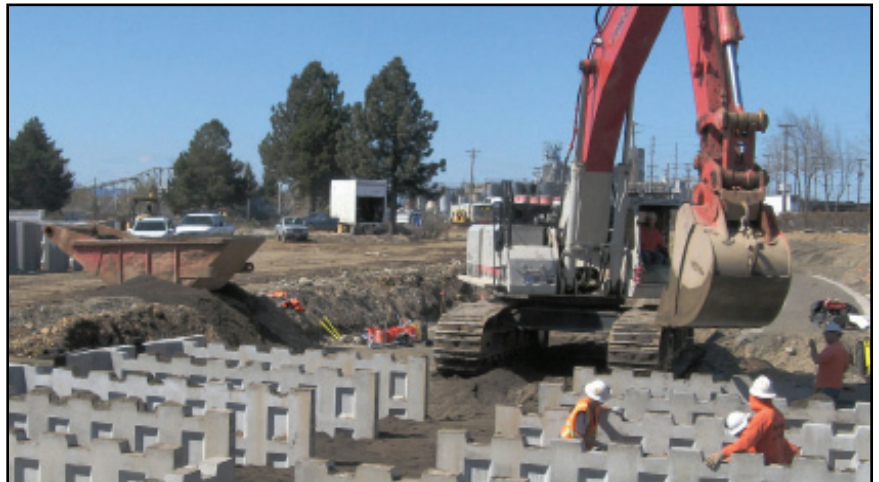
Excavator – back-to-back walls
