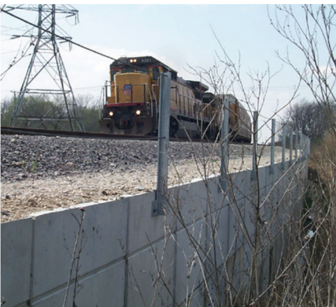
HAND-RAIL POST INSTALLED ON WALL FACE:
