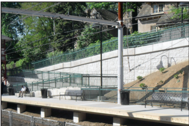
HAND-RAIL POST INSTALLED ON WALL FACE:
