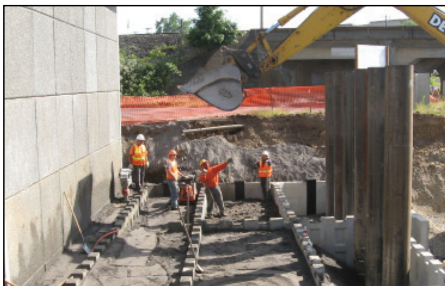
Excavator with reversed bucket
