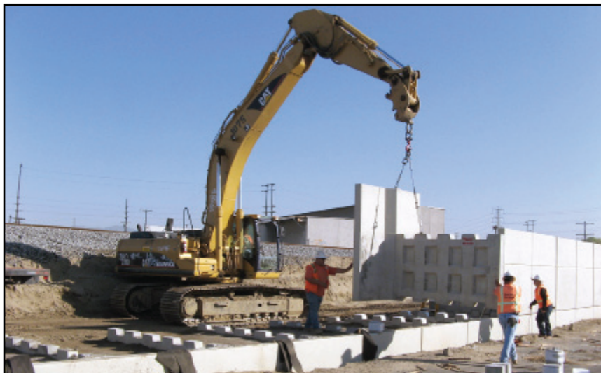
Excavator with slings - working behind the wall
