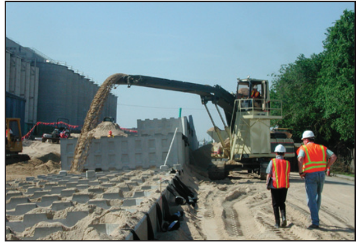
Placing the backfill
