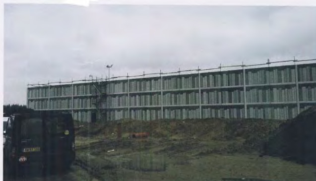
New building under construction in Viborg in Jutland
