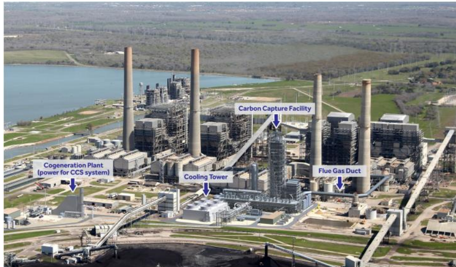
圖 7 NRG Energy Parish CCS project
