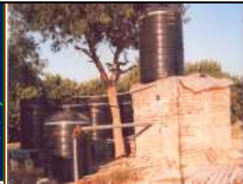
Set up for preparing different quality water for drip irrigation
