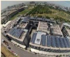
Fig 6. Photovoltaic Panels installed on roof top to generate electricity, save costs and reduce CO2 emission.
