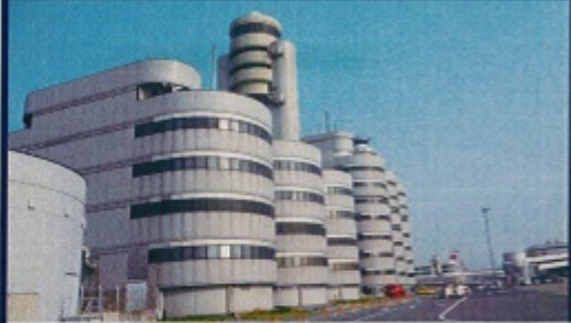
New Administrative Building
