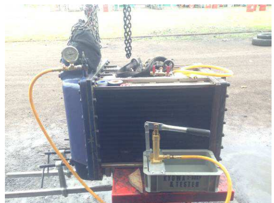
Air Cooler 試壓
