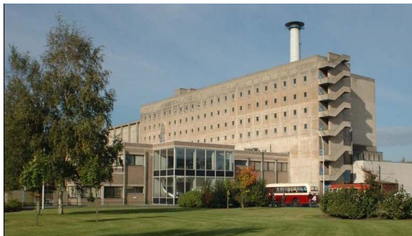
Eurochemic Reprocessing Plant 除役前外觀
