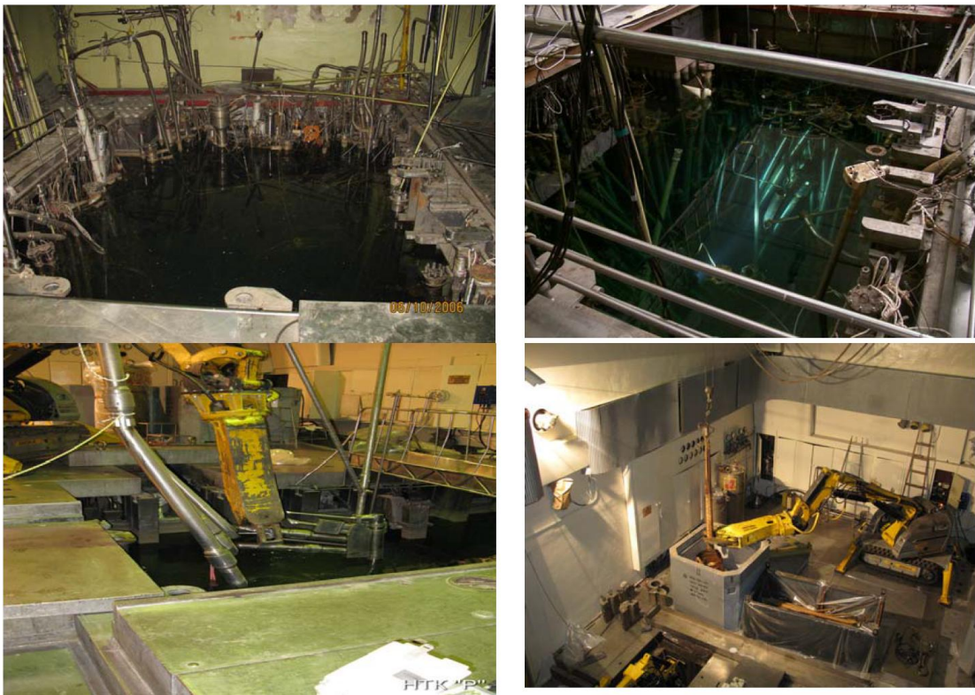
Fig. 3. Removal of loop channels from the reactor pool.
