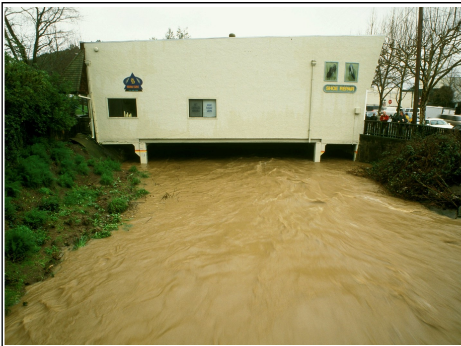
'Building Bridge 2' in San Anselmo seriously restricts high flows in San Anselmo Creek. The Town's water level gauge is located beneath the building. Photo by Charles Kennard
