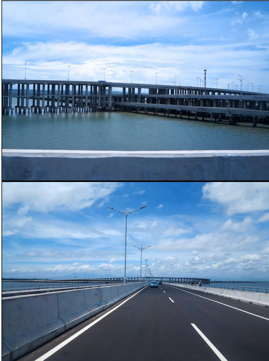
Bali Mandara Toll Road & Expressway
