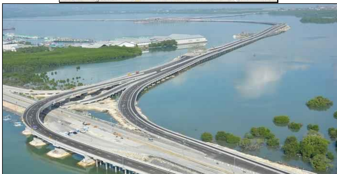
Bali Mandara Toll Road & Expressway 5
