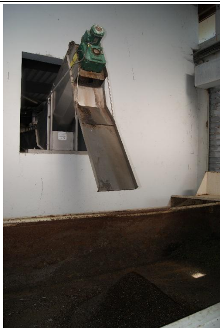
氣曝浮除沉砂後之砂礫
