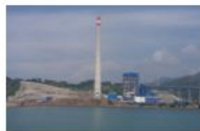
UBOH Banten 1 Suralaya Steam Coal PP 600 MW (O&M)
