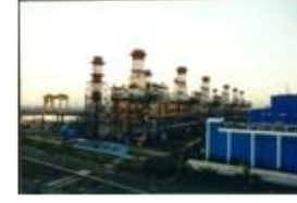
UP Semarang CCGT & SPP 1,469.16 MW
