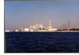
UP Priok GT, CCGT & Diesel PP 1,348 MW
