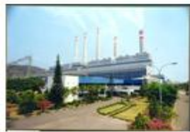
UP Suralaya Steam Coal PP 3,400 MW
