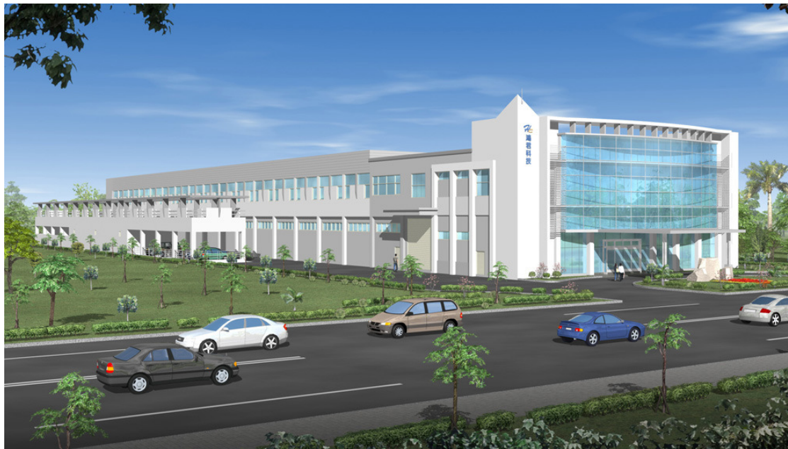
Figure 4: The blueprint of the new factory of Hung Chun Bio-S Co., Ltd.
