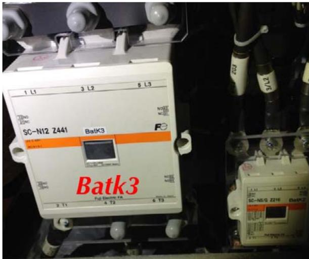
3. 第 11 號線：110V battery (135AH) B101 (+) →BatN1 (5A) NFB for BatK→102→HCRN (5A) NFB for Head Car Control→120→key start up
